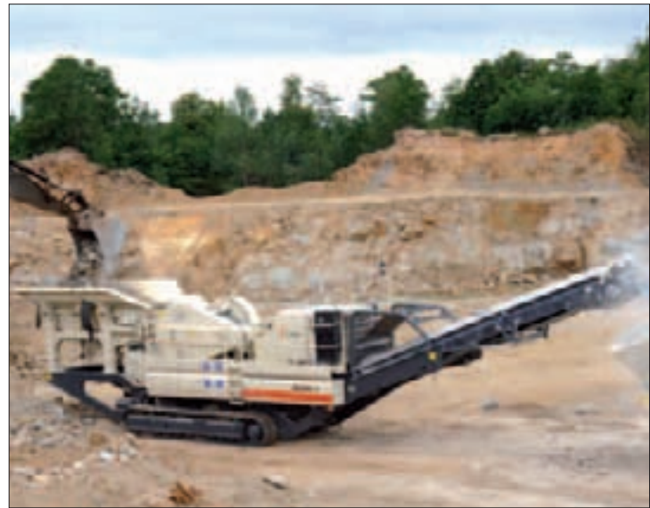
Primary crushing of blasted aggregates with LT116 in Poland.
