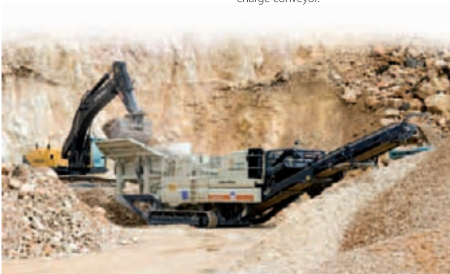
Contract crushing with the Lokotrack LT1213 in Spain.
